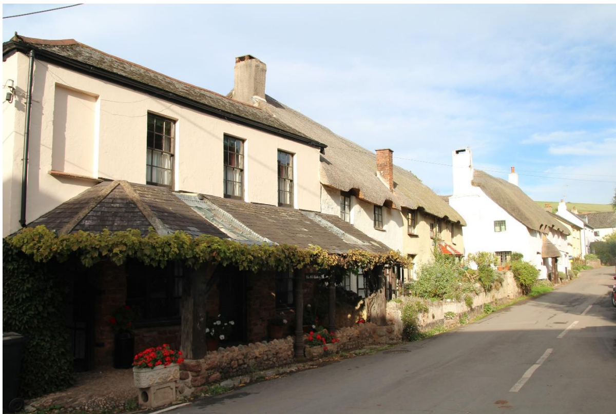
View of vernacular cottages in Stokeinteignhead with cob and thatch, and stone and slate, painted white and cream.
